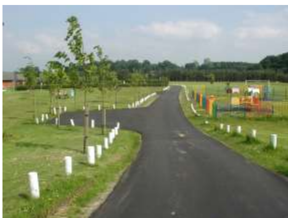
Above: New driveway, play equipment and trees at Mainsforth Sports Complex
